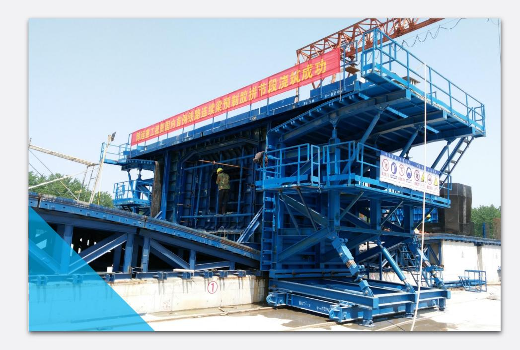
Segmental assembly formwork system is applied to precast cantilever segmental assembly girder. It is new style non-standard equipment. We have launched BY1507 Automatic precast segmental box girder formwork system with the advantages of less land occupation, easy to operate, less restricted by topography, easy beam plant layout, high utilization for formworks and pedestal and shortened the construction period greatly.
