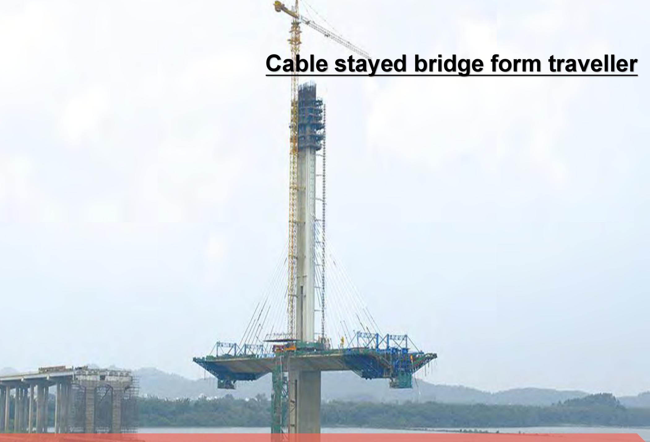
The Yingde Bei Jiang three bridge is located in the Yingde City of GuangDong province. The length of the bridge is **4.27 kilometers**, and the main spans of Bei Jiang Cable-Stayed Bridge are **160m+160m** single tower and single cable plane and pier tower girder consolidation, single box girder 3 section and total investment of the project is nearly 400 million RMB. The project completed in 2016.
